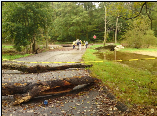
Damage Assessment teams comprised of officials from FEMA, PEMA, and the County evaluate damage to a culvert in Hopewell Township.
