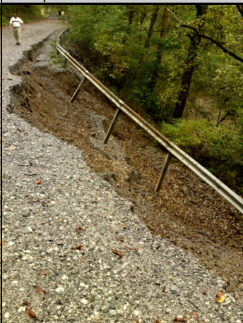
Collapsed road near Glen Rock.
