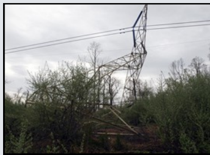
High tension lines toppled during an EF2 tornado at Ski Roundtop: 4-28-11
